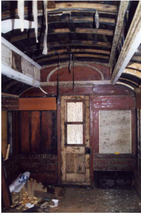
After stripping the paint at the men's saloon area.
